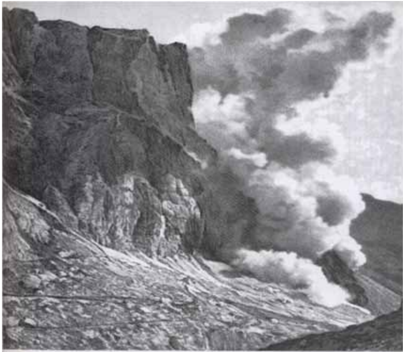
The demolition of the Italian rock ledge at the small Lagazuoi on 22 May 1917. Picture taken by Major Karl von Raschin first Imperial Infantry Regiment five minutes after the explosion.
